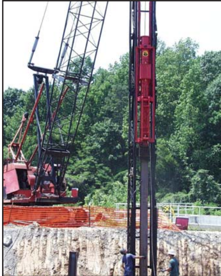
D19-42 driving H-beam.
